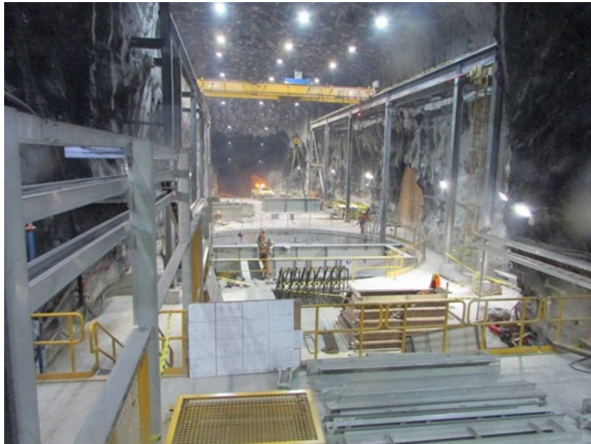
Freeport Underground Mine, sheave deck installation, Indonesia
