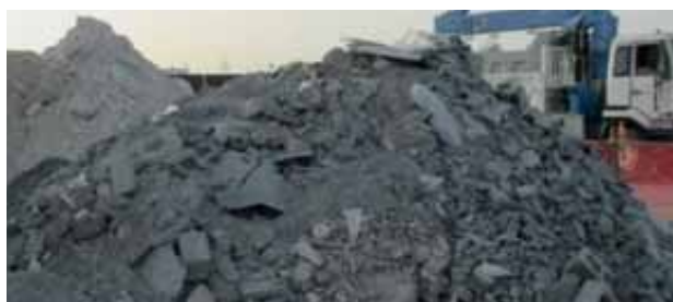
CONCRETE RECOVERED FOR REUSE AT TECH 4, QATAR.
