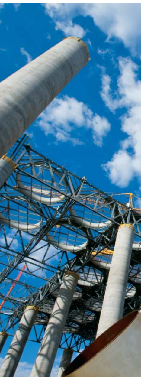
Medupi power station air cooled condensers
