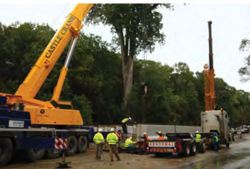
Installation of bridge beams at the Storms River Bridge
