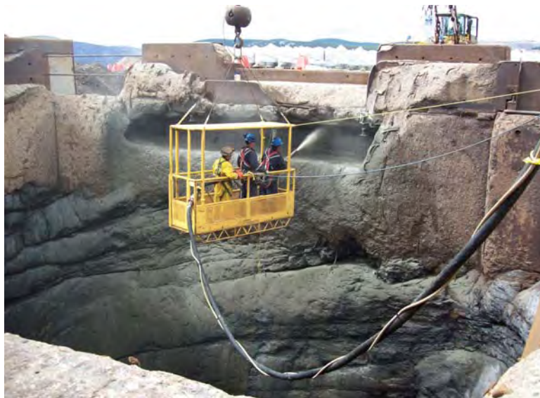
Shotcreting open pit truck dump at the Iron Ore Company of Canada's mine near Labrador City
