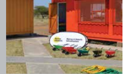
Murray & Roberts Infrastructure Concor Karena Joint Venture Medupi Power Station Reabetswe Village Construction of new creche
