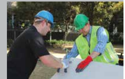
Murray & Roberts Infrastructure Noupoort Wind Farms Noupoort Village Repairs to damaged roofs of 50 households
